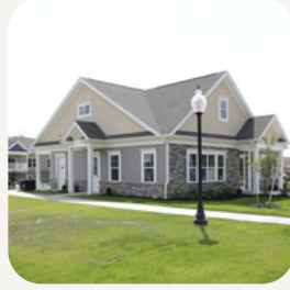
East Pointe Apartments
